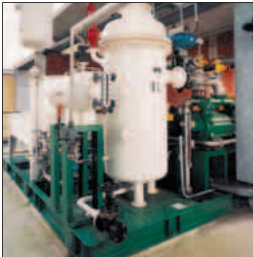
Fig 42: Liquid ring vacuum pump on a chemical plant
